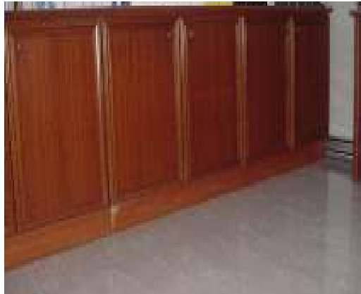
Item Low cabinet overall size 3000mm x 550mm x 760mm with veneer ply and nyatoh timber edging and skirting c/w door in natural stains lacquer
